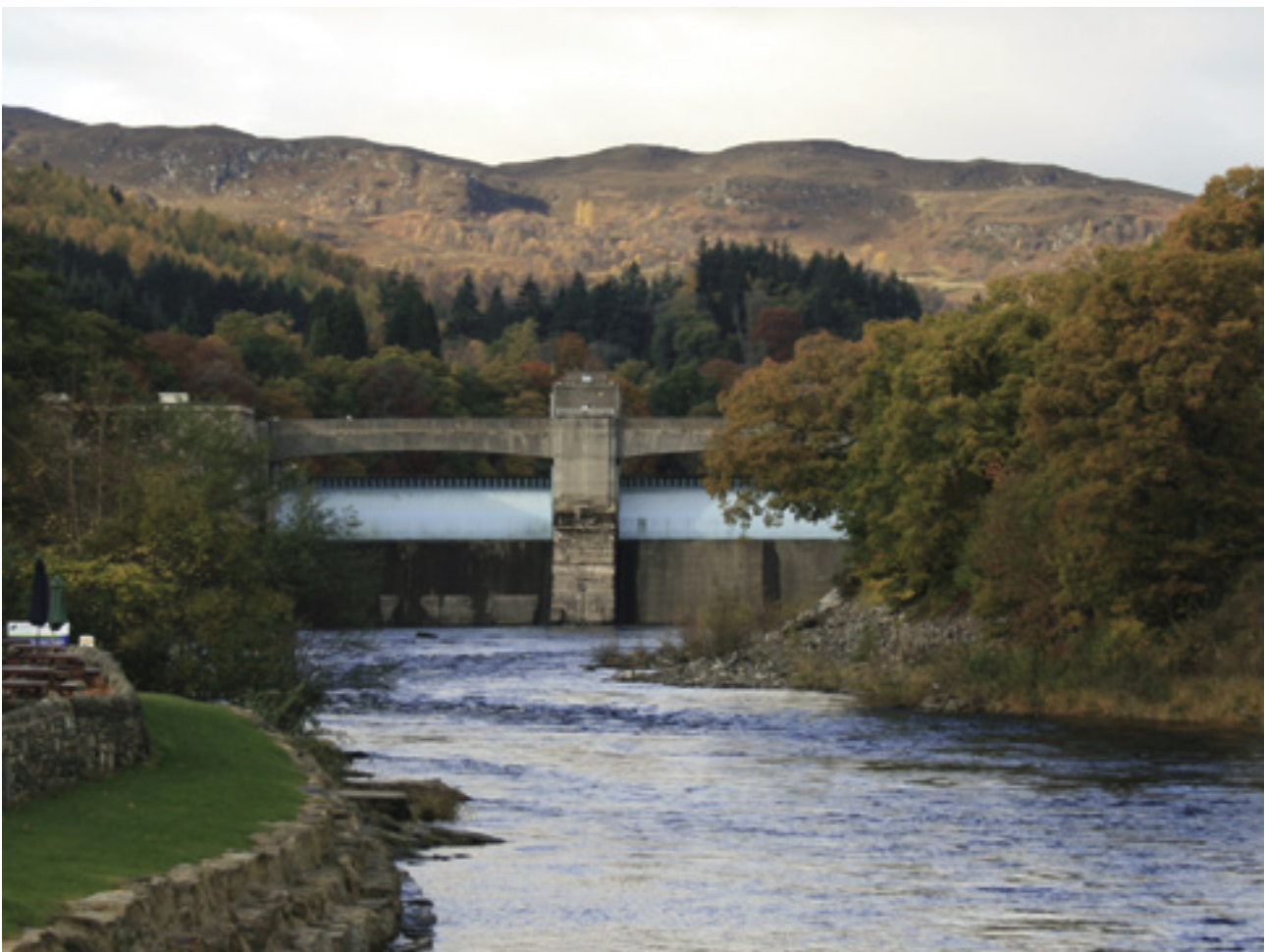
Pitlochry hydroelectric power station
