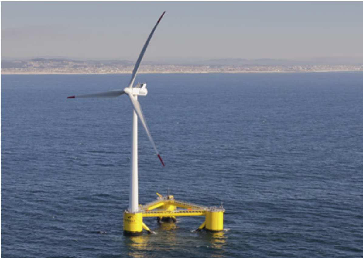
A floating wind turbine – image courtesy of Principle Power
