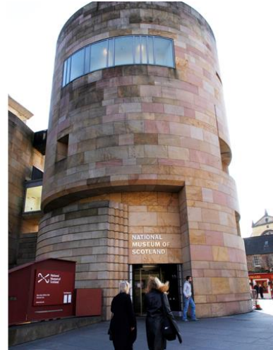
The Tower Entrance
